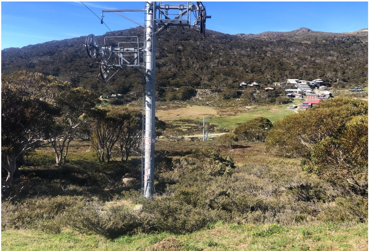
Photo 2: Access to Tower 2 and Tower 3 will require 1-2 excavator movements from Kosciuszko Road down the existing lift alignment.
